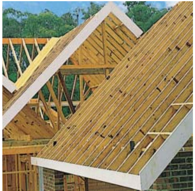
Long length Hyspan rafters for house under construction at Eltham, Victoria.
